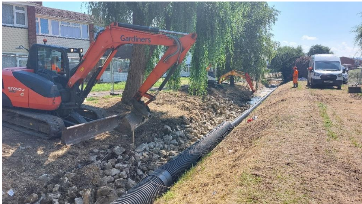
During works - removal of concrete channel
