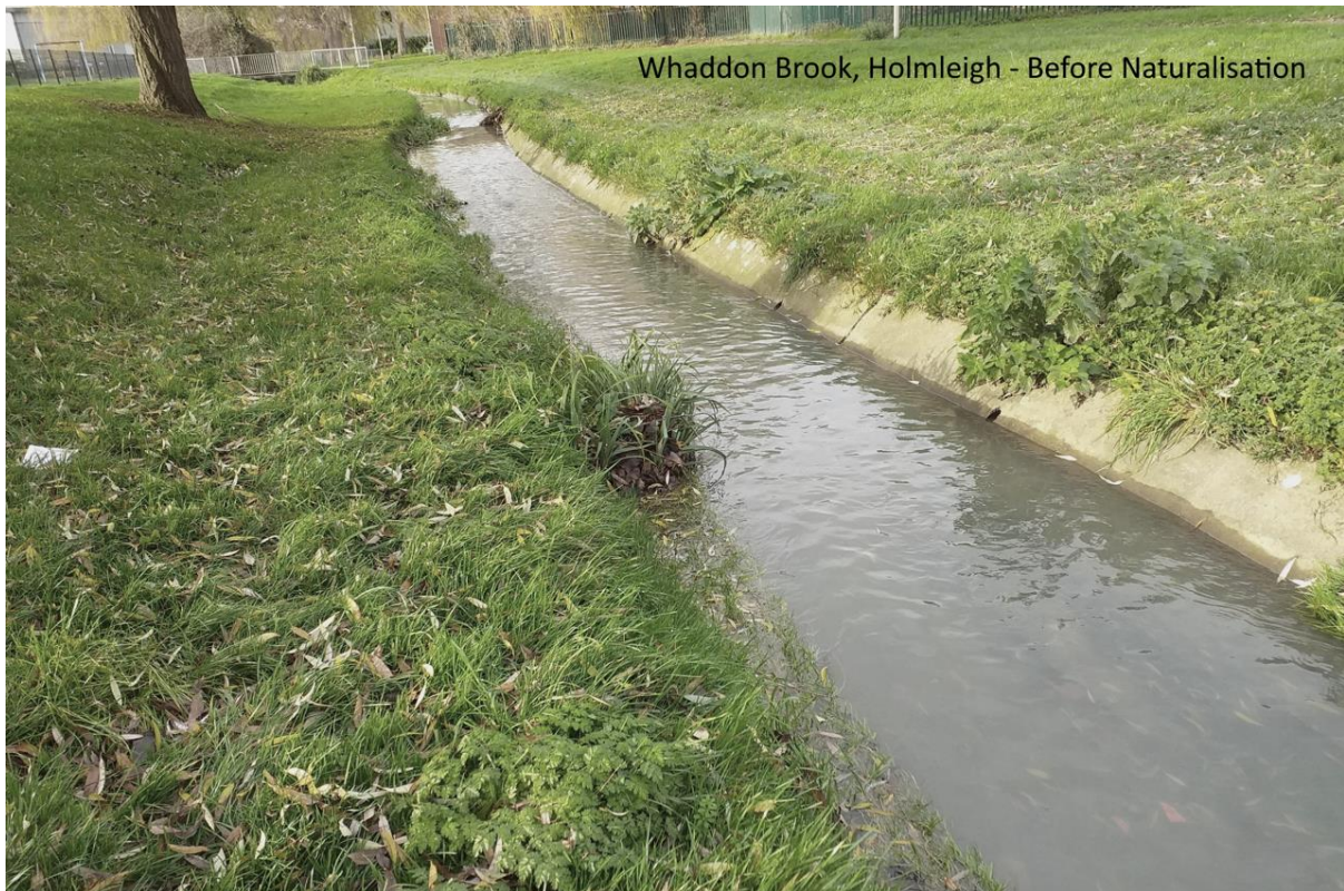
Prior to work - a barren concrete channel, with very little biodiversity
